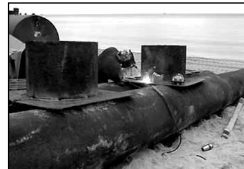
Worker welding 30" pipe for carrying sand to the beach
