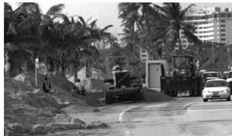
Salvaged sand piled up along A1A being returned to Ft. Lauderdale Beach
