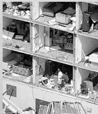
Wind penetration eviscerates condo wall
