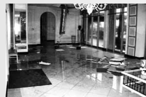
Boarded up windows in disheveled Plaza East lobby
