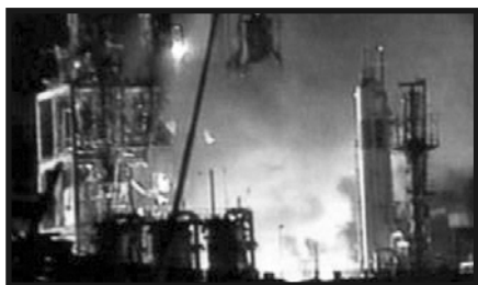
(Aftermath of the 2004 Skikda, Algeria LNG Disaster)
