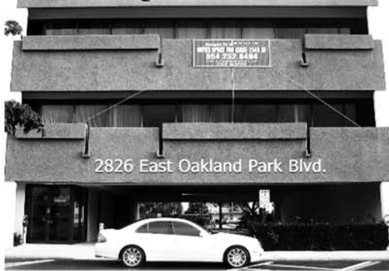
OAKLAND PARK BOULEVARD JUST EAST OF BAYVIEW DRIVE ON THE SOUTH SIDE OF THE ROAD
