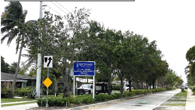
NE 6th Ave Drainage Project
